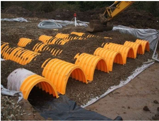
Figure 27: StormTech Storm Storage Tank
