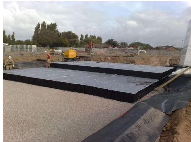
Figure 28: StormCell Storm Storage System
